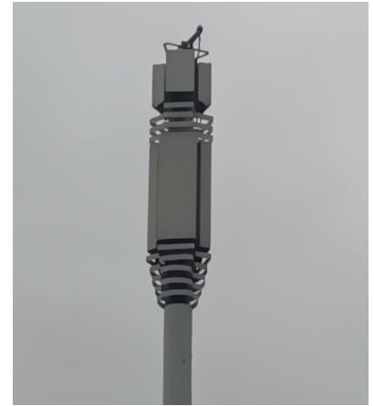
One of three signal towers along a stretch of the A610 and residential, Nottingham.
